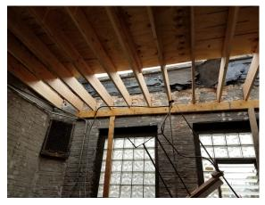
Replacement of collapsed roof, walls and bowstring trusses on a 100 plus year old building. Project included shoring and remediation of remaining existing trusses, repair of bowed brick walls and existing membranes to new structural wall supports and installation of new trusses.
